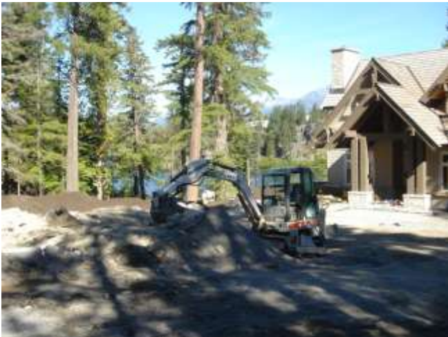
Work progress Summer 2006:
