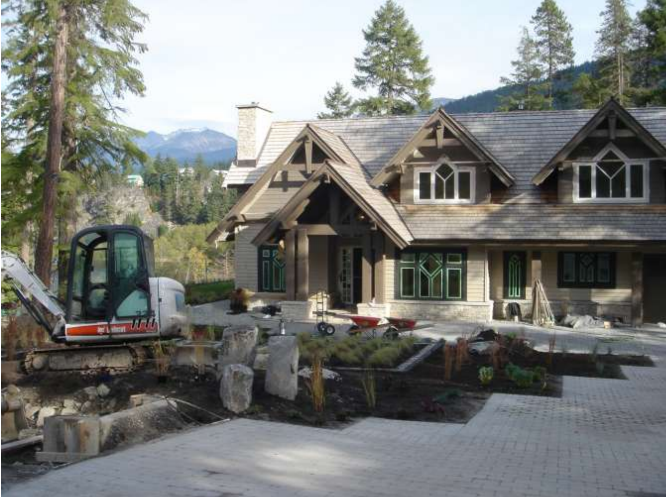
Under construction 3: Basalt columns – Front berm – Details:
