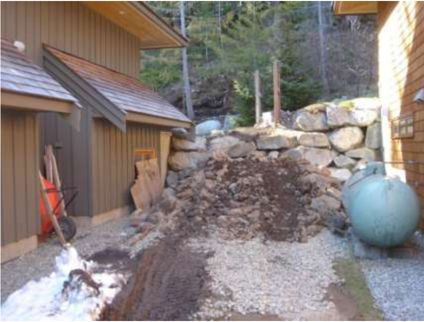
Photo 8 – Alpine project – Before
