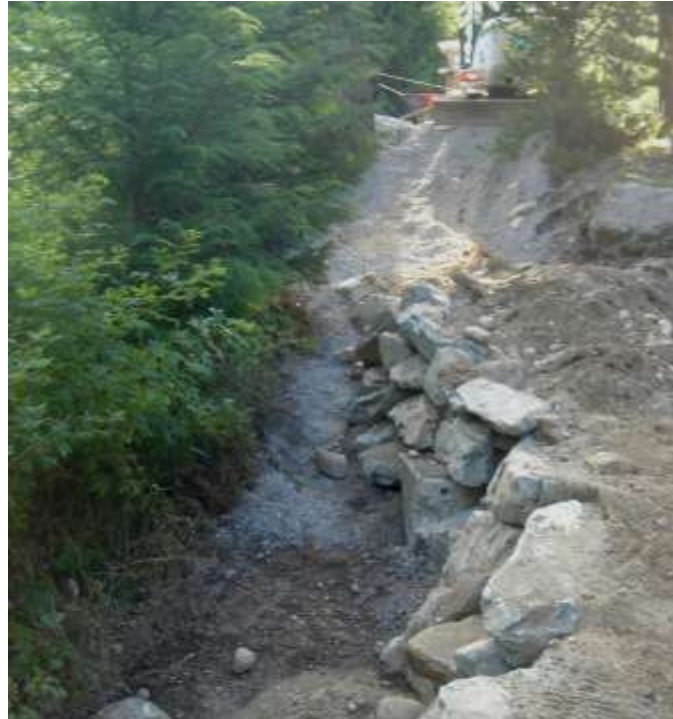
Back Yard - Under Construction – Retain. Wall:
