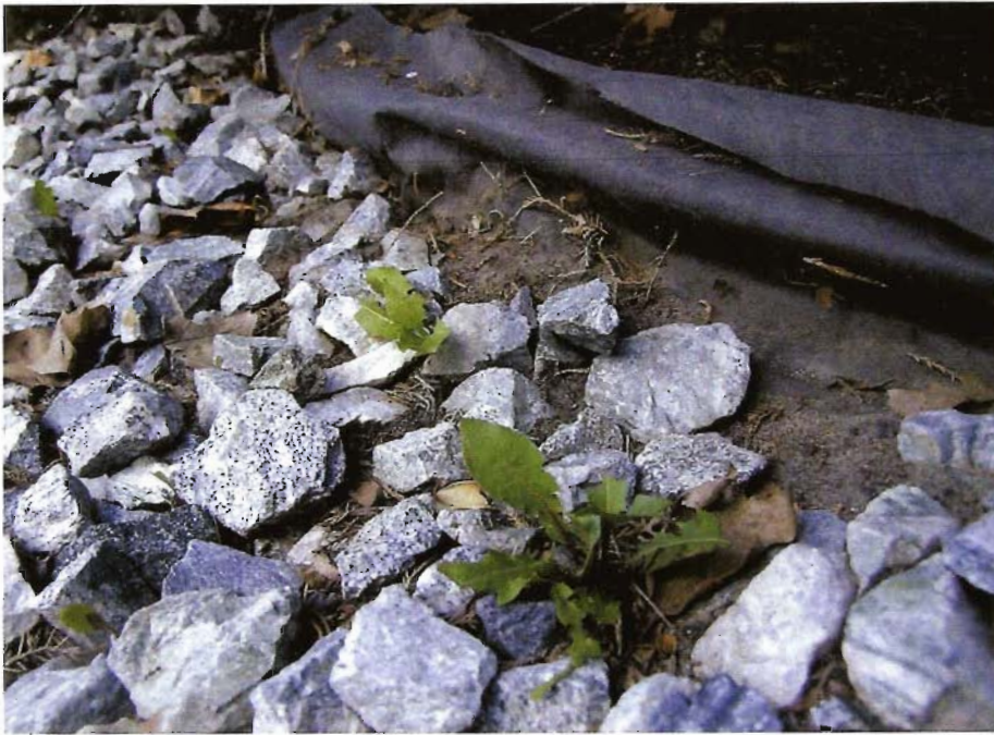
Soil naturally accumulates between the rocks on top of fabric so dandelions and other annual weeds will have a nice place to germinate.
