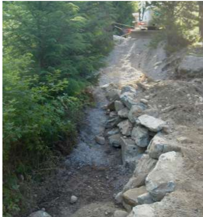
Back Yard - Under Construction – Retain. Wall:
