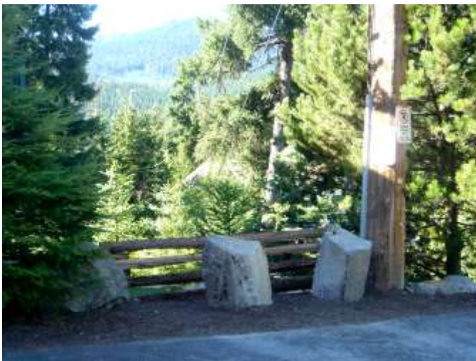
View from Road after Construction:
