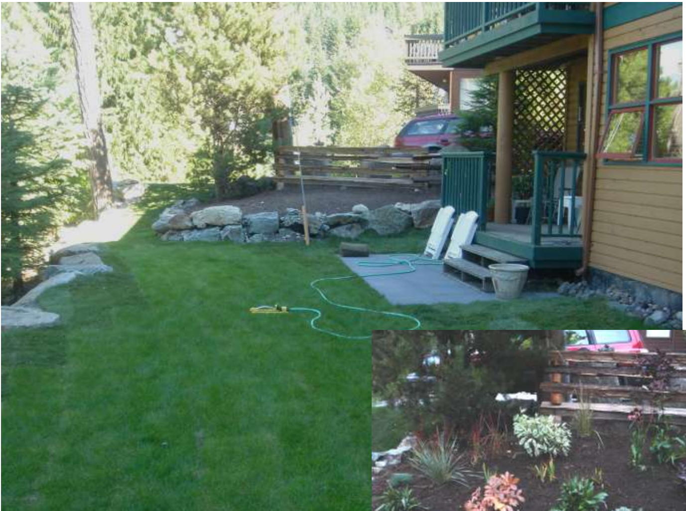
After: – Lawn and garden bed installed: (Planting to finalize project, see small picture below:)
