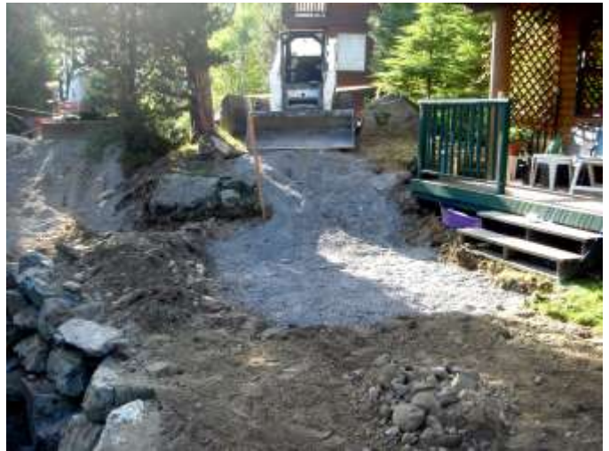
Under Construction: Access for excavator:
