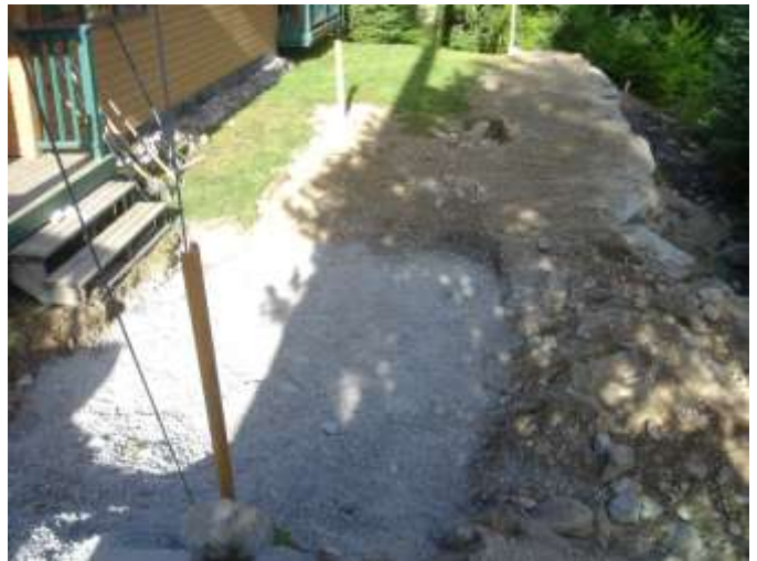
Under Construction 1: Retaining Wall and Fill.
