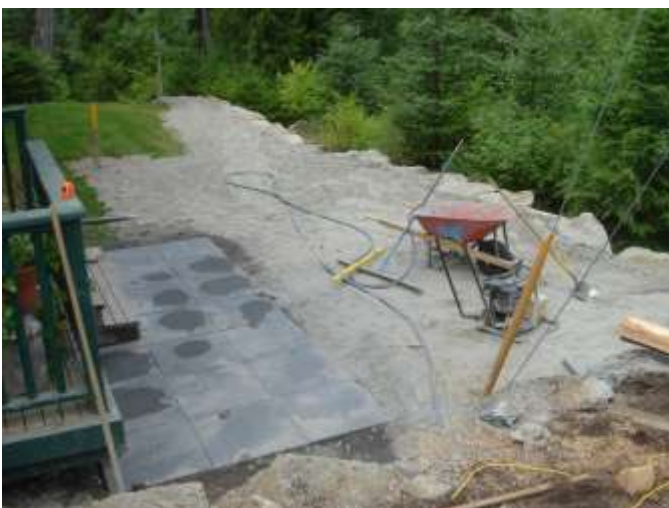
Under Construction: Patio, Grading.
